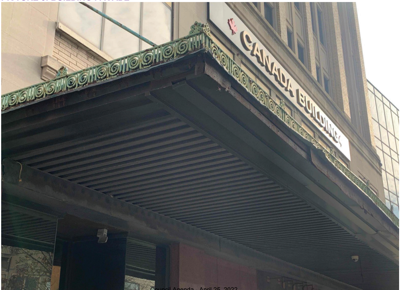
PICTURE 5: BUILDING FACADE
