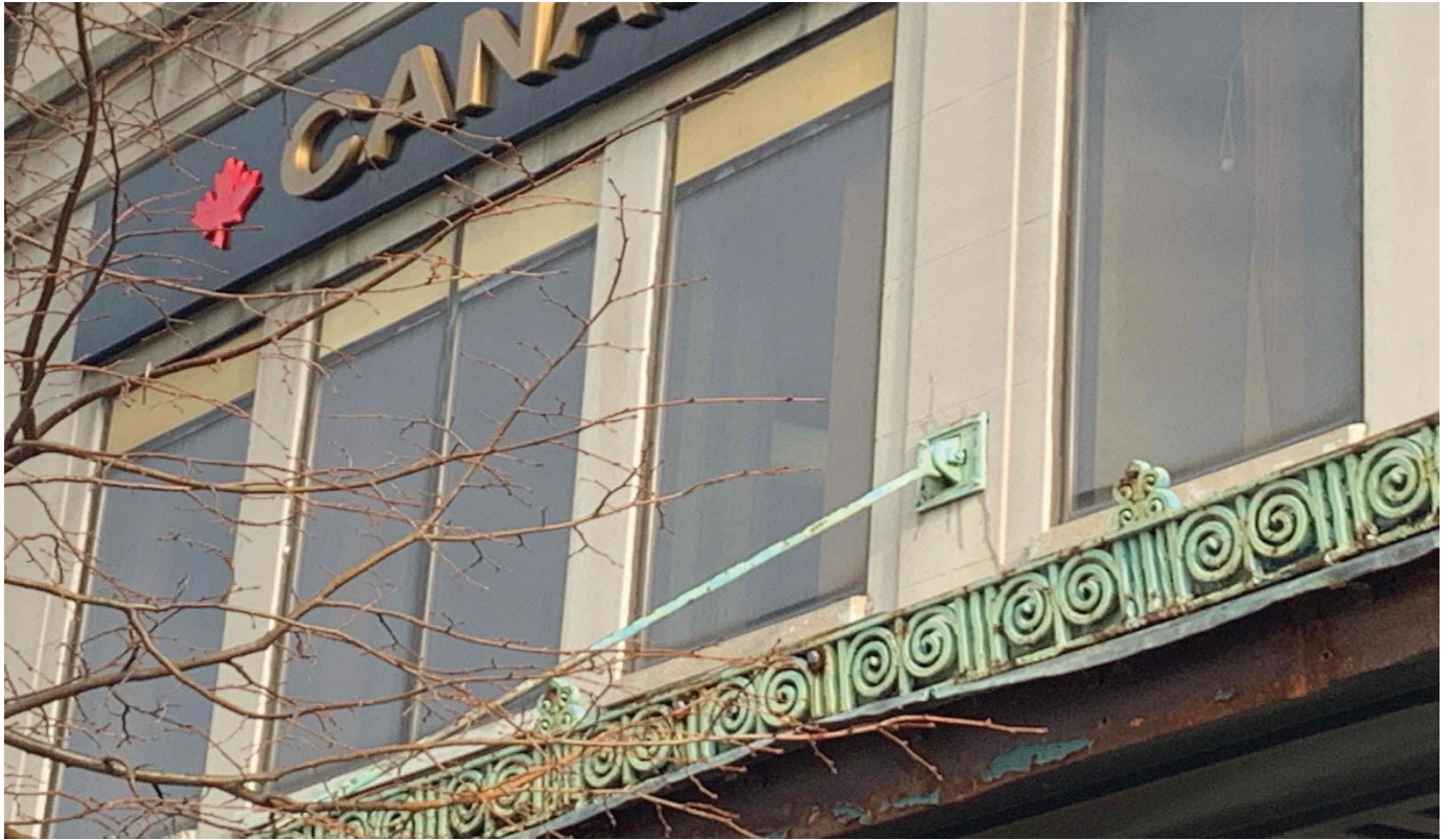
PICTURE 4: BUILDING FACADE
