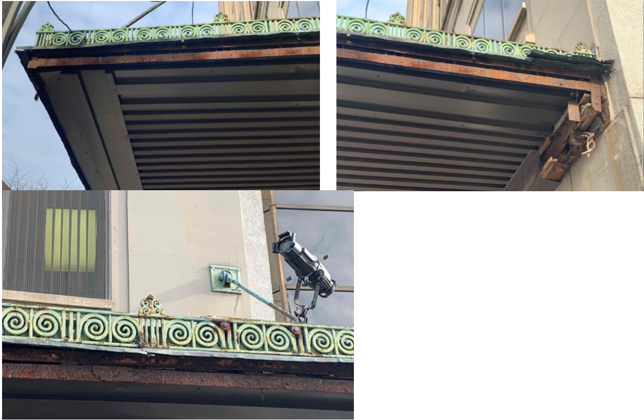
Photographs of existing canopy and decorative trim
